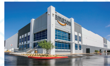
Amazon Data Center
